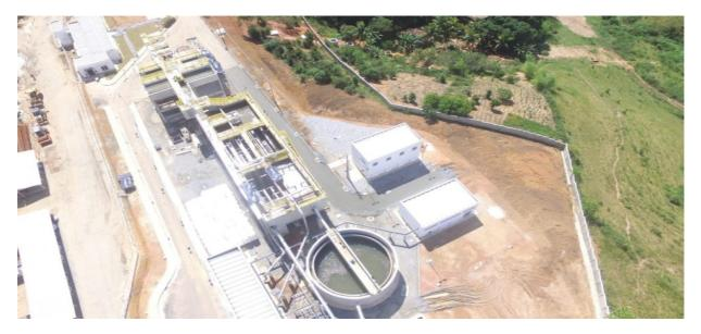
In 2017 Biowater Technology AS through local partner Memphis Empreendimento proposed CFIC<sup>®</sup> as the solution for the wastewater treatment. This technology was chosen over other technologies as UASB, Activated Sludge, MBBR and IFAS due to its advantages including compactness, low TSS in the effluent (no need for a separate separation stage), ease of operation, and low operational cost.
