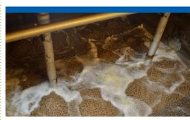
CFIC® reactor contains highly packed biofilm carriers to a degree (typically 90-99% bulk volumetric fill) that little movement of the carriers occurs in the reactor during normal operation.
